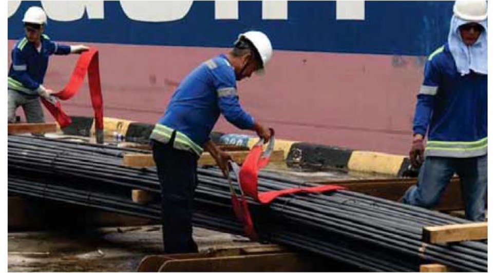
✔ Pre-slinging of two tiers of rebar in preparation for loading
