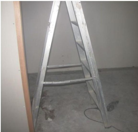
Figure 1: The workers were working on the A-Frame ladders when they lost their balance and landed on the concrete floor
